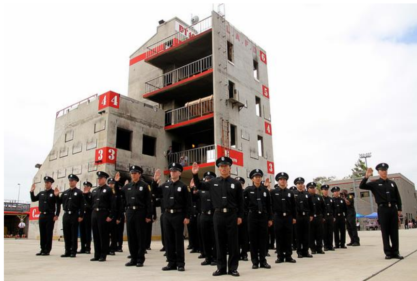
LAFD DRILL TOWER 40 San Pedro
